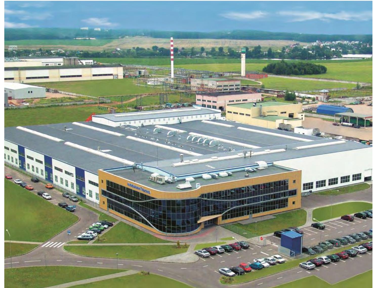
AluminTechno, LLC Production Facility
